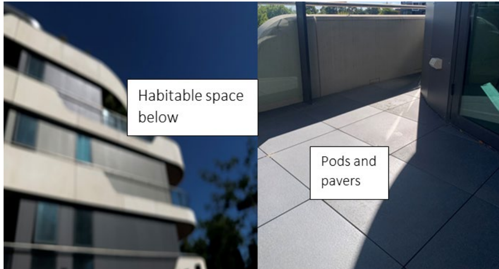
Figure 75: Case Study E - balcony construction
