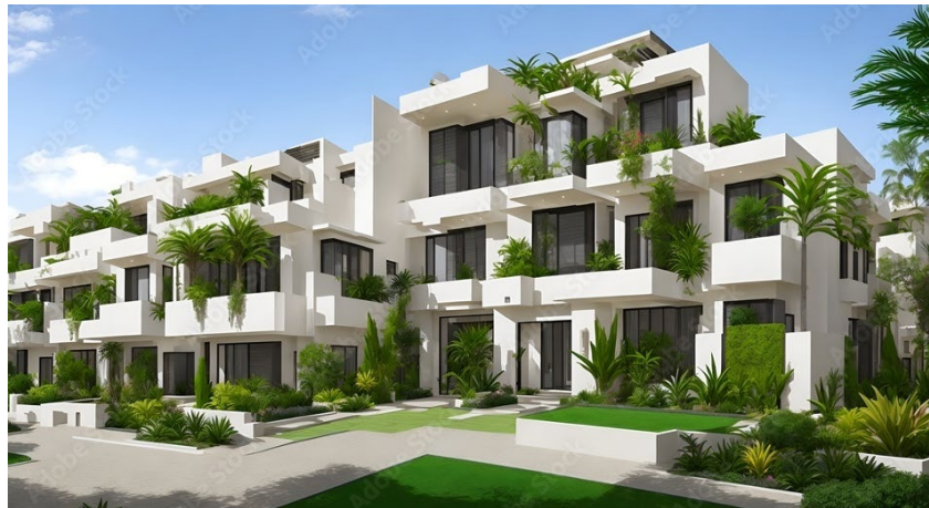
Figure 22: Balconies with plants, presenting the potential for heavy loading issues
